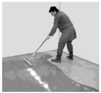
6. The floor spreading tool is used to smooth out the surface after it has been raked or spreading the poured cement if the surface is too irregular to use the thickness rake.
