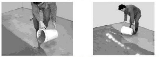
Pour the smoothing cement whilst walking along, and always apply to the wet working edge.
