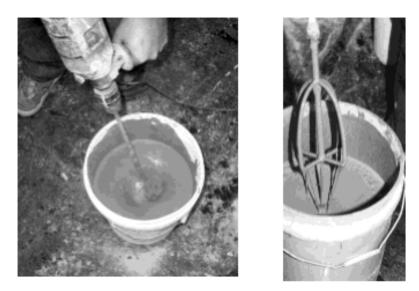
After mixing the smoothing cement should be smooth and free flowing. Note – Do not add water more than the recommended amounts as this can seriously affect the performance of the material.
